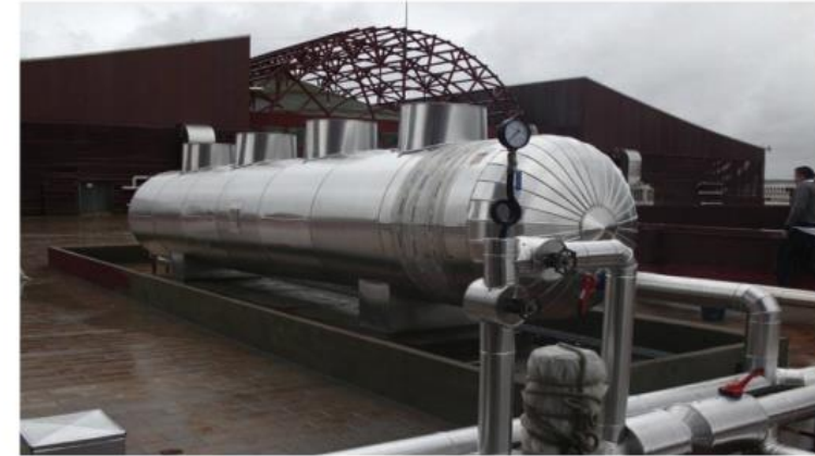
Fig. 19. Storage tank implemented in a real solar cooling installation at the University of Sevilla (Spain) |
