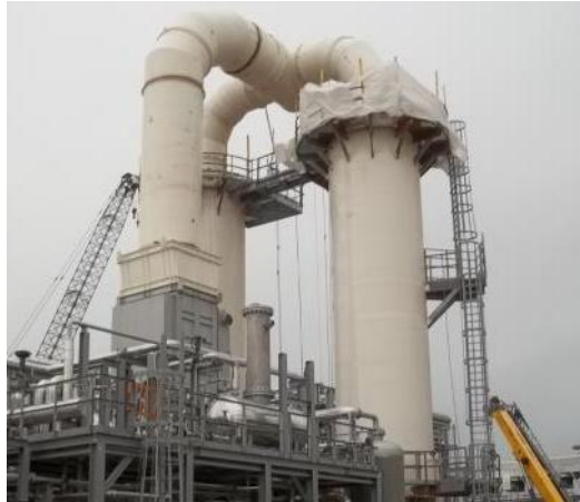
Steam methane reformer
