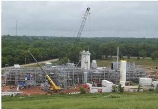
View of GTL plant from landfill site
