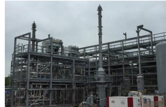
LFTL and HFTL columns
