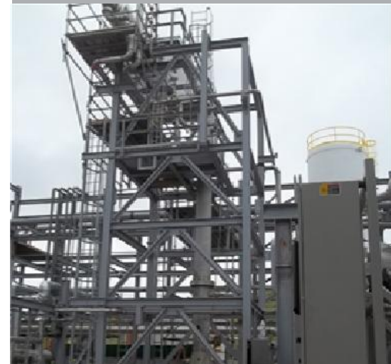
CO 2 wash column
